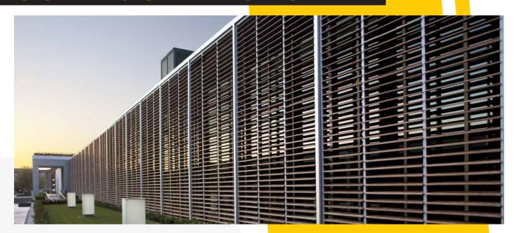
Metal Craft Sun louver system is a highly functional, yet architecturally pleasing system that can add color and exciting design effects to a building facade. The system is available with panel set at the range o angles and wide range of colors and size. Also, Metal Craft sun louver system provides for flexibility in design, easy maintenance and fast installation.
