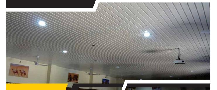
Finish of the tiles: Tiles are available in plain and perforation of 2.5 mm and 1.7 mm
